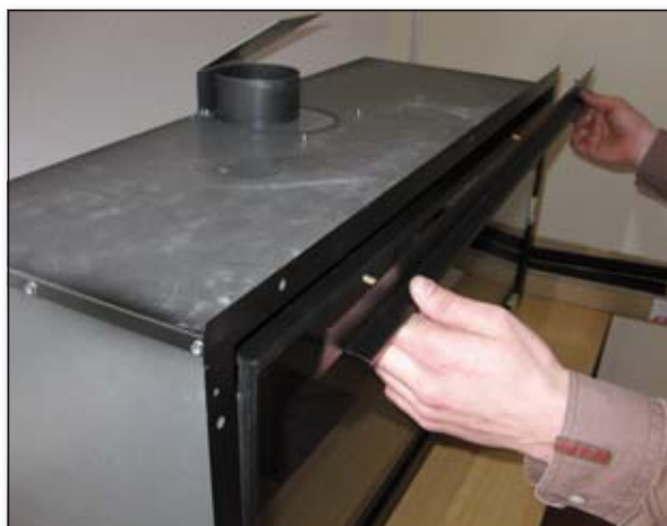
In case of frameless first mount the 4 profiles of the plaster trim
