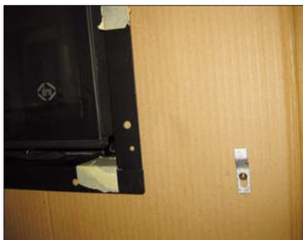
Bèta frame only: drill 4 holes and mount brackets on the drilled holes (see included installation sheet)
