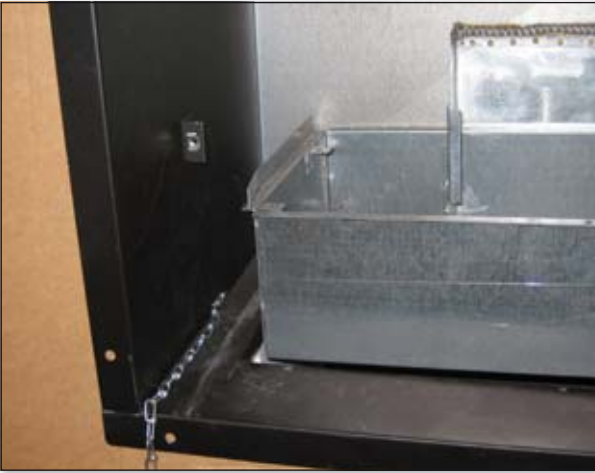
Mount gas control box to convection box
