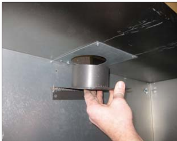
Place flue spigot in top of convection box (in case of flue liner no debris shield)
