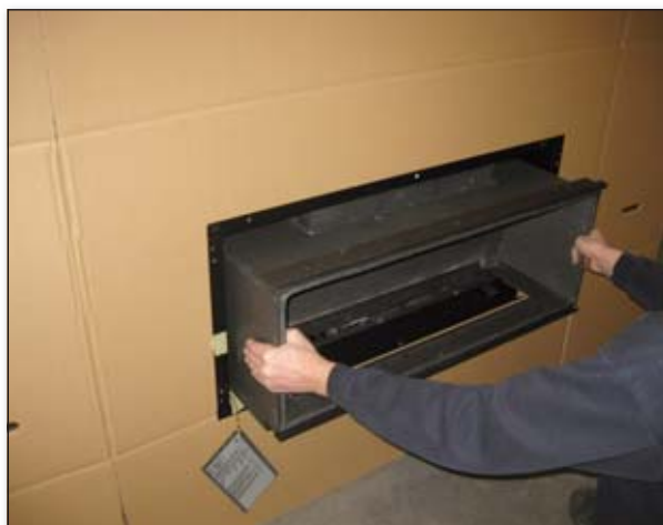
Slide combustion chamber into convection box
