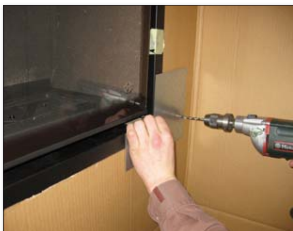
Bèta frame only: use the drilling jig to mark 4x drill spots (see included installation sheet)
