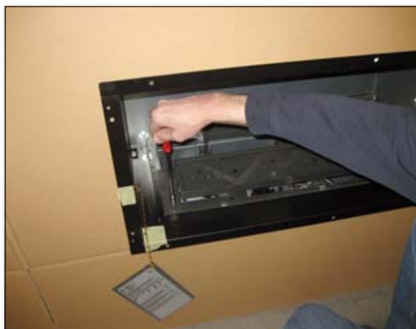
Fix burner with screws (which were removed before)
