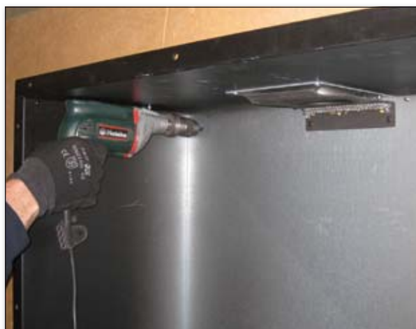
Mount the convection box to the wall (see installation manual for disassembling the appliance)
