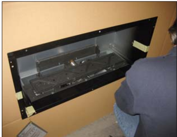
Place burner in convection box
