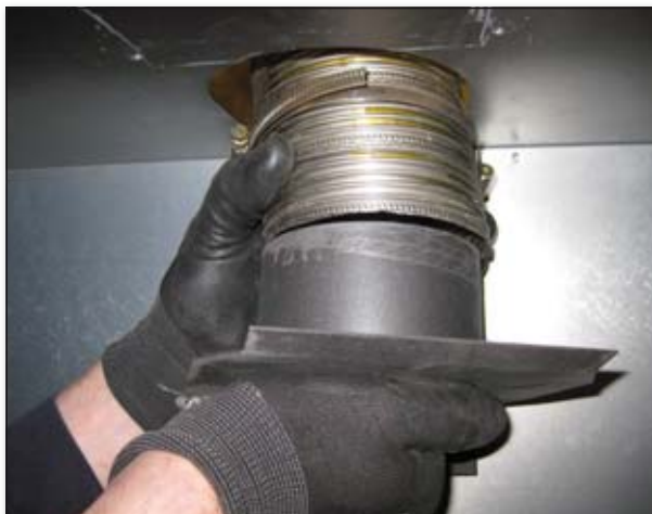
Mount flex flue line in flue spigot (flue liner only)
