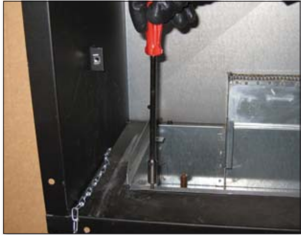
Mount gas control box to convection box
