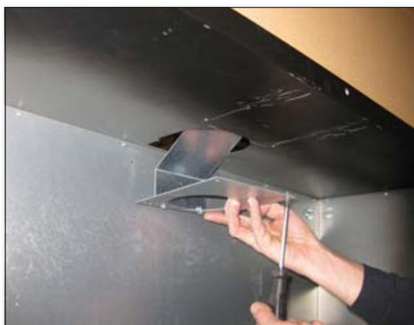
Place debris shield (linerless application only)
