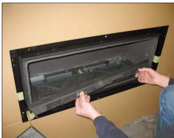
Put vermiculite tray in place
