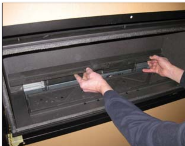
Put vermiculite tray in place
