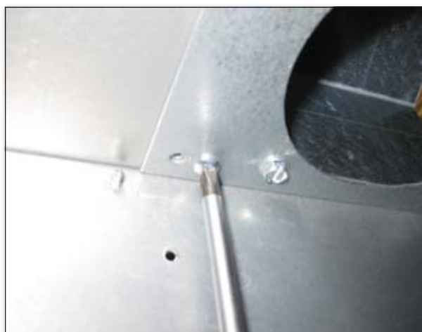
Use the inner holes (Linerless application only)
