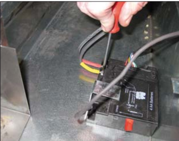
Connect the receiver to gas control (Global 90 CF)
