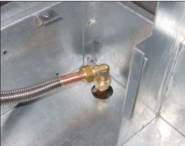
Connect the flexible gas pipe to the gas supply with an elbow
