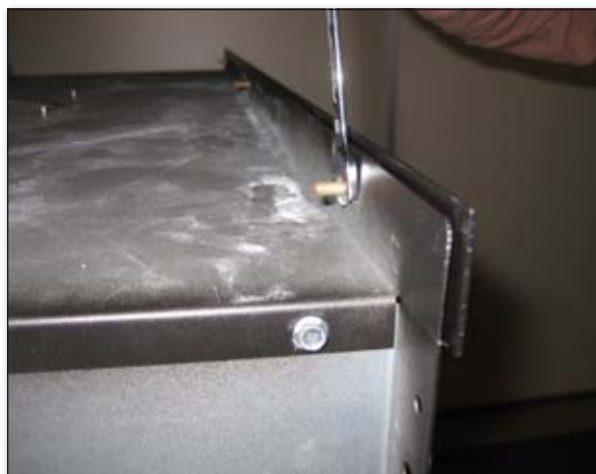
Profile with spoiler on top. The studs should be in the center of the hole!
