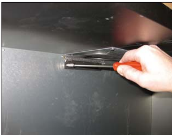
Mount flue spigot with 2 screws
