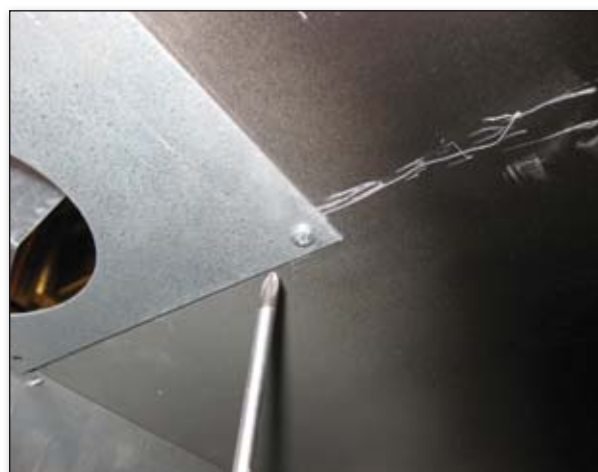
Use the flat topped screws (Linerless application only)
